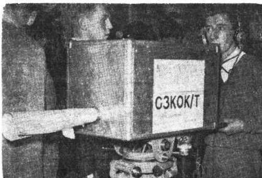
BIG STUFF Brian Partridge G3KOK/T operates the Image orthicon camera at the 1956 Convention. The lens hood was an afterthought - and that tripod head cost 10/- scrap!
